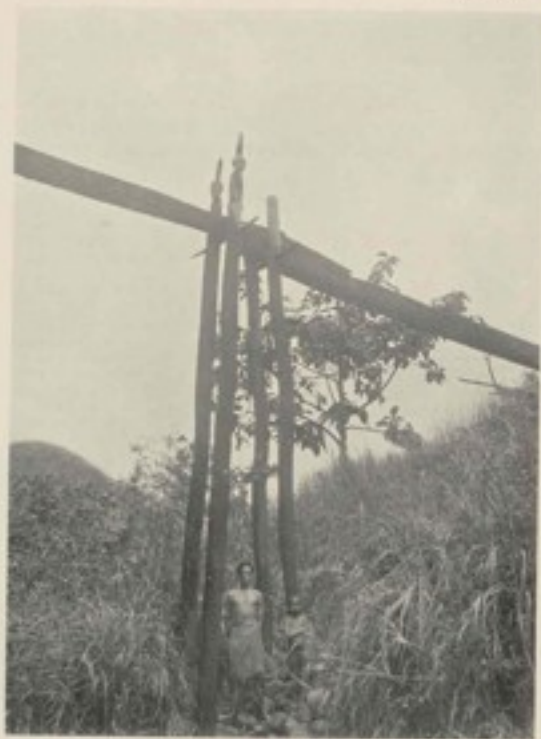
Aqueduct across the Davao creek (Bartle Bay) showing carved figures on posts
